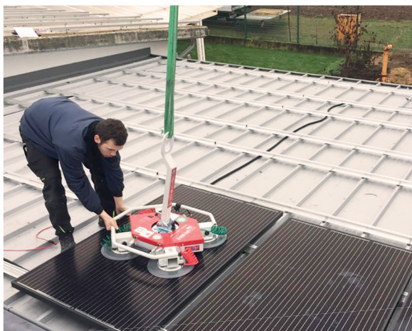
The UPG350 can suction elements such as solar panels, veneered wood, metal and plastic panels and much more
